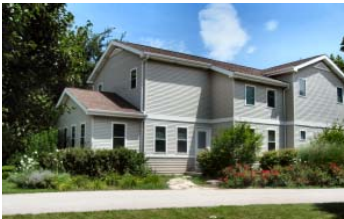
The YMCA Network runs a transitional housing project at a residence
